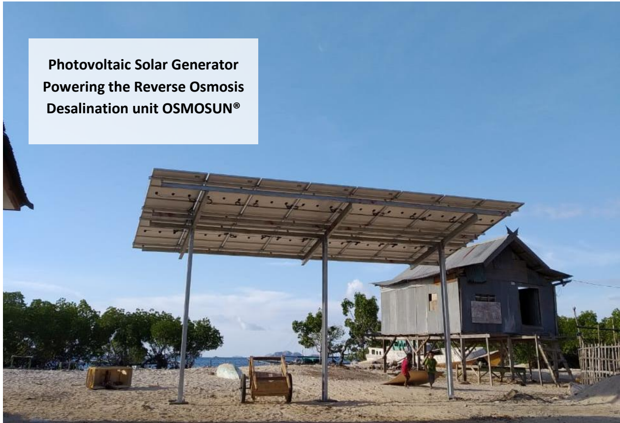
Drinking water daily production of 5m 3 powered by 100% solar energy
